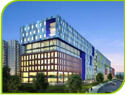
VRV units Kidwai Nagar Revamp
